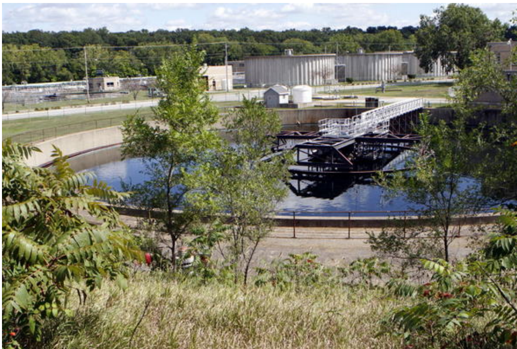
City of South Bend Wastewater Treatment Plant
